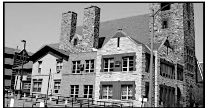
The stone façade on the front and side of 227 N. Capitol today.
