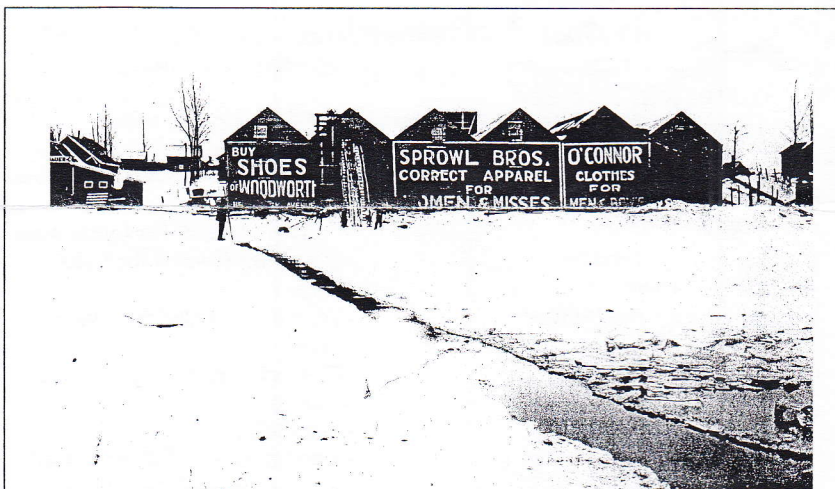
The Clear-Bauer Company cutting 'up river' ice just west of the Logan Street Bridge and on the south bank of the Grand River in 1917. Prior to the advent of the icemaker and refrigerator, ice for the home was cut from the river to allow the storage of goods that would spoil if not kept cool. In the center of the photograph the conveyor for moving the ice from the river and into the storage sheds is visible. The ice would be packed in sawdust and straw and last until September or October. Why was it called up river ice? Well many people believed that prior to sewage treatment it was better to cut the ice up river of the city. The Pure Ice Company purchased the Clear-Bauer Company in 1920. FPML/CADL.
